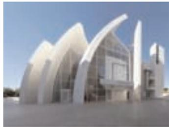
windows, where the coating of titanium dioxide, along with sunlight, catalyses the breakdown of the dirt landing on the
